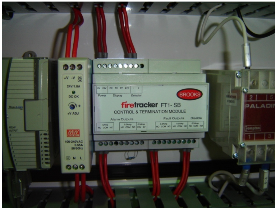
Figure 8 Control / Termination Module & Power Supply mounting
