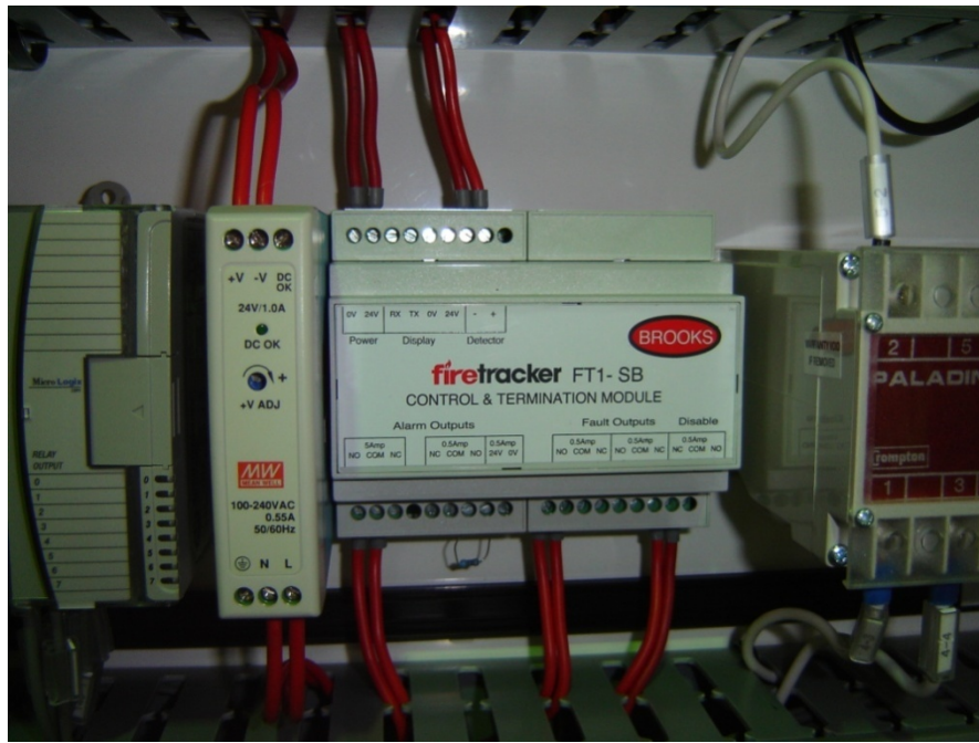
Figure 7 Control / Termination Module & Power Supply mounting
