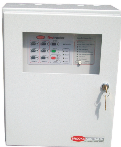
Figure 14 Gas Extinguishing Control Panel
